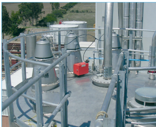
Stainless steel modular bin vents
